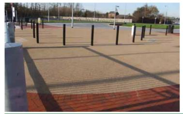
NOTE: A suitable steel, wood, brick, stone or aluminium edging should be provided to ensure a neat edge detail.
